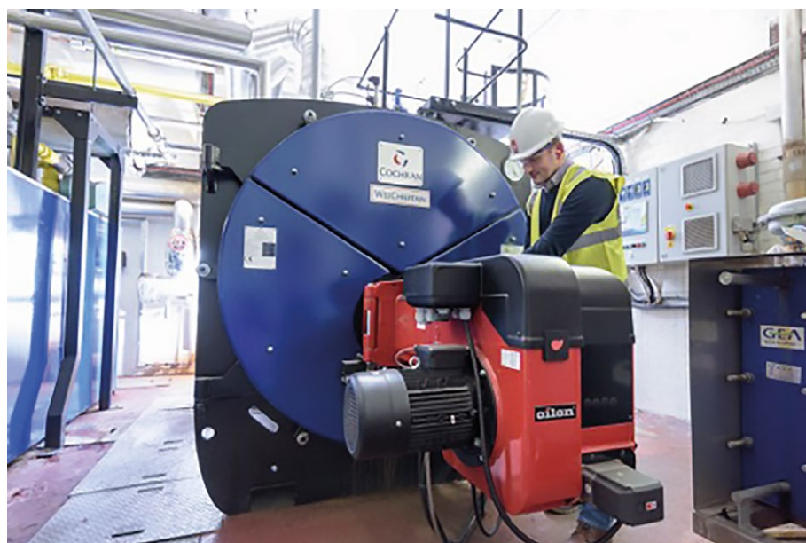
A regular burner service ensures the efficient and reliable operation of a boiler through its lifecycle.
