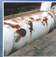
VISIBLE CORROSION ON EXPOSED STEEL
