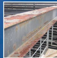
VISIBLE CORROSION ON EXPOSED STEEL
