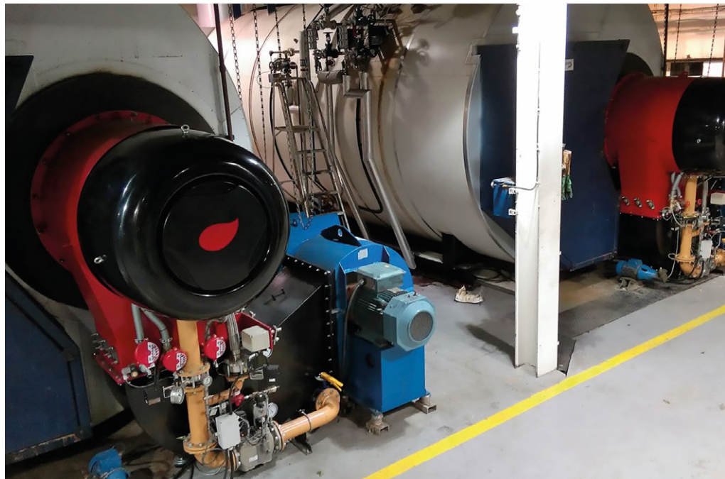
A new burner allowed a turndown of 8:1 at a hygiene product manufacturer, improving efficiency at low firing rates.
