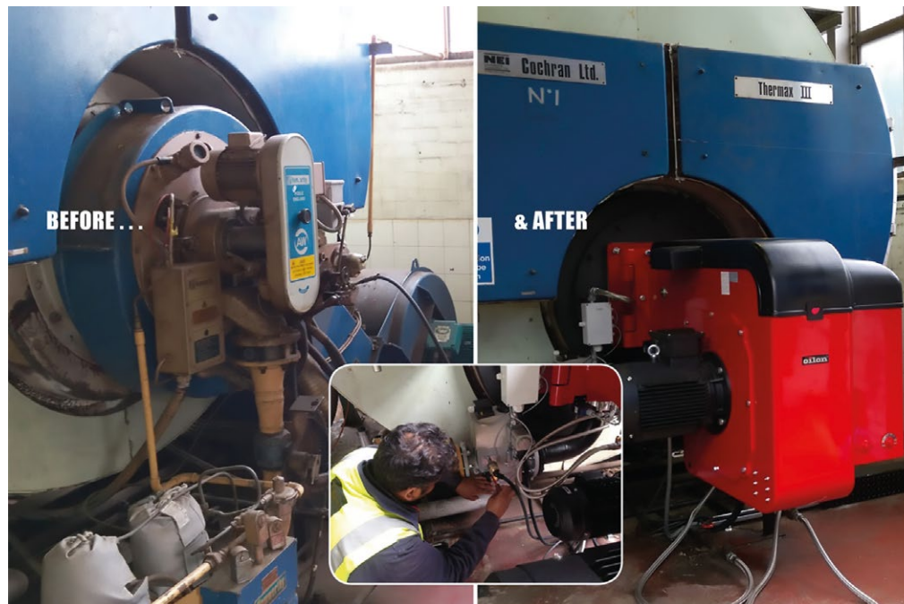
For a food manufacturer, a new burner with digital combustion control and energy saving equipment including an economiser reduced fuel use by nearly 13%
